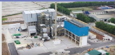
Waste to Energy Plant (Vietnam) JFE Engineering Corporation
